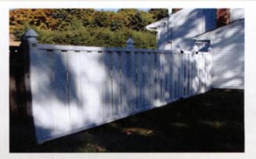
THE MIRAGE (SHADOWBOX) -1 x 6" vertical boards -3 1/2" x 3 1/2" rails
